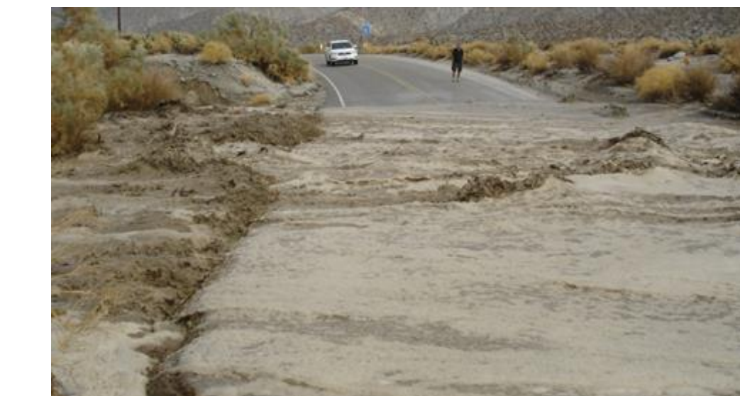
Figure 7: Flooding across Highway 78 in San Diego County, California, 22 Jul 2013. [Photo credit: NOAA]
