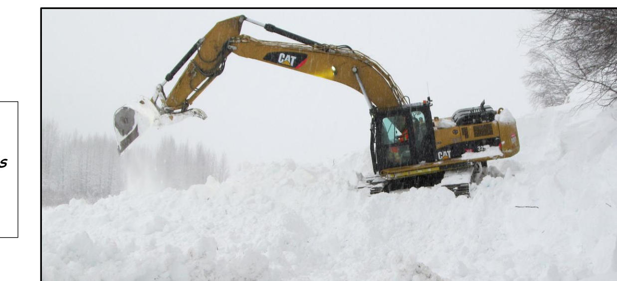
Right: Heavy equipment works to dig out buried train cars and clear the tracks during a multi-day closure after an avalanche. Photo courtesy of Alaska Railroad.
