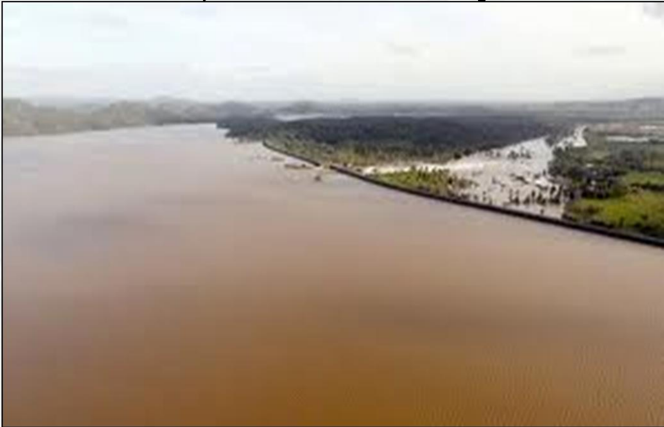
Wivenhoe dam and reservoir (almost filled -1.9 MAF)
