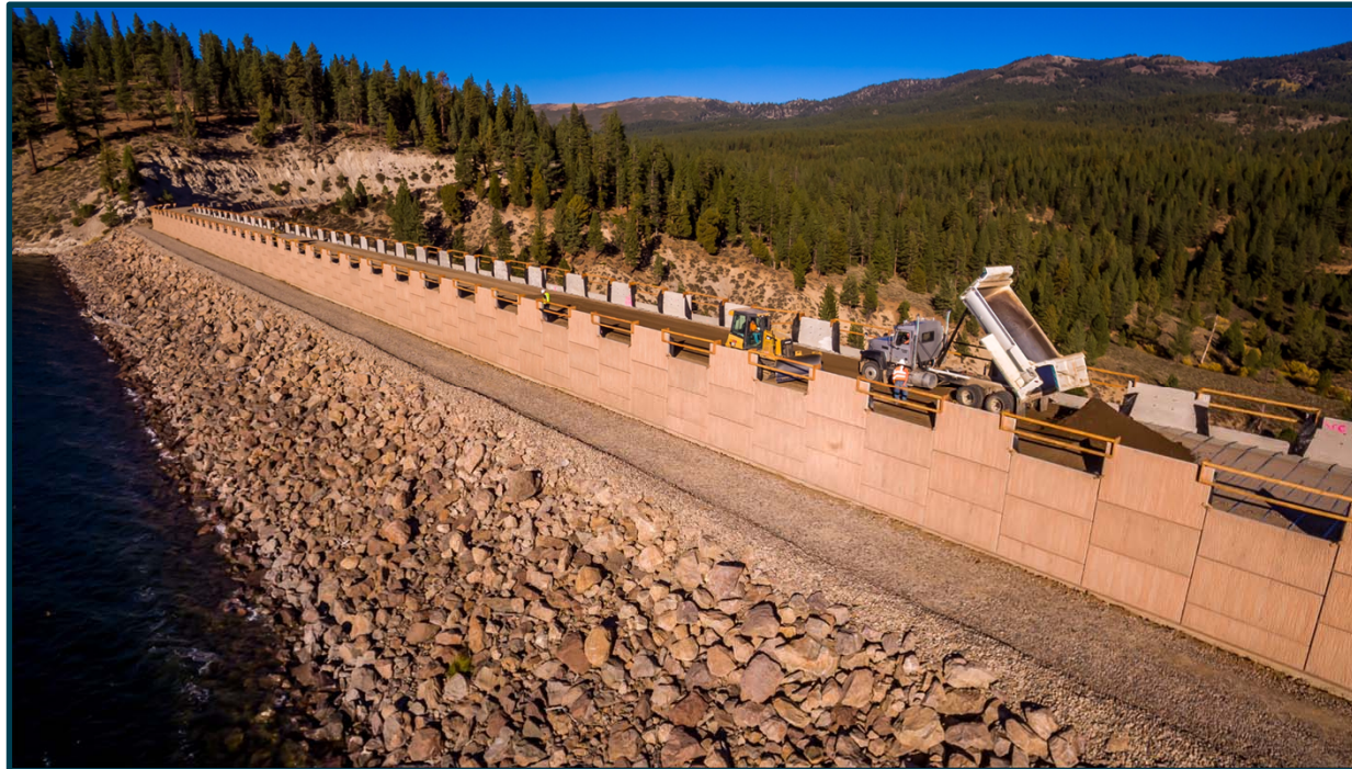
Construction of a Mechanically Stabilized Earth (MSE) wall at Stampede.
