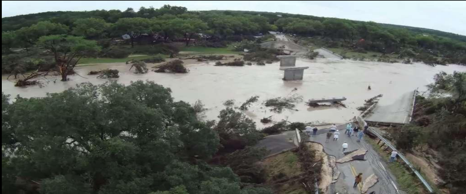
Fischer Store Bridge Memorial Day flood of 2015
