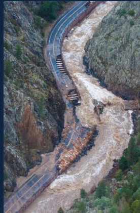
2013: Big Thompson Canyon (~7500 ft) washed out US 34 in floods
