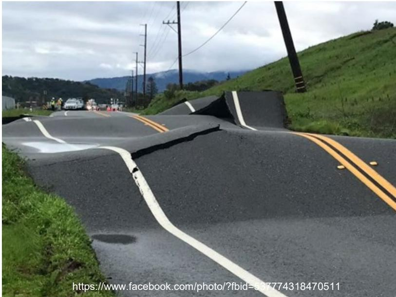
Severe damage was caused to a roadway in Marin County due to a hill slope failure, resulting in buckling of the road
