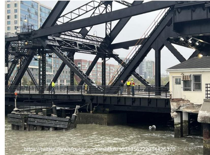
Strong winds and high surf caused multiple barges to break away from moorings and drift into the Third Street Bridge in San Francisco, causing damage to the structure
