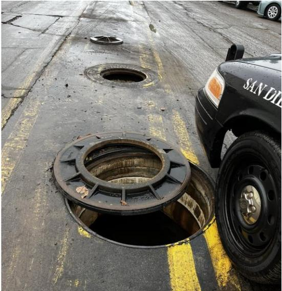
**Manhole covers over stormwater drain pipes were lifted from their position as floodwaters overwhelmed drainage**
