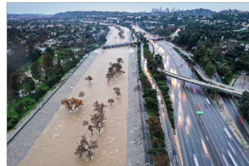
High Flow through the Los Angeles River
