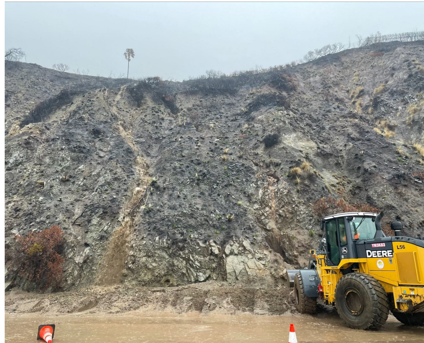
Debris flows onto the Pacific Coast Highway (left) and material covering Topanga Canyon Boulevard after a significant debris flow, both within the Palisades Fire Burn.
