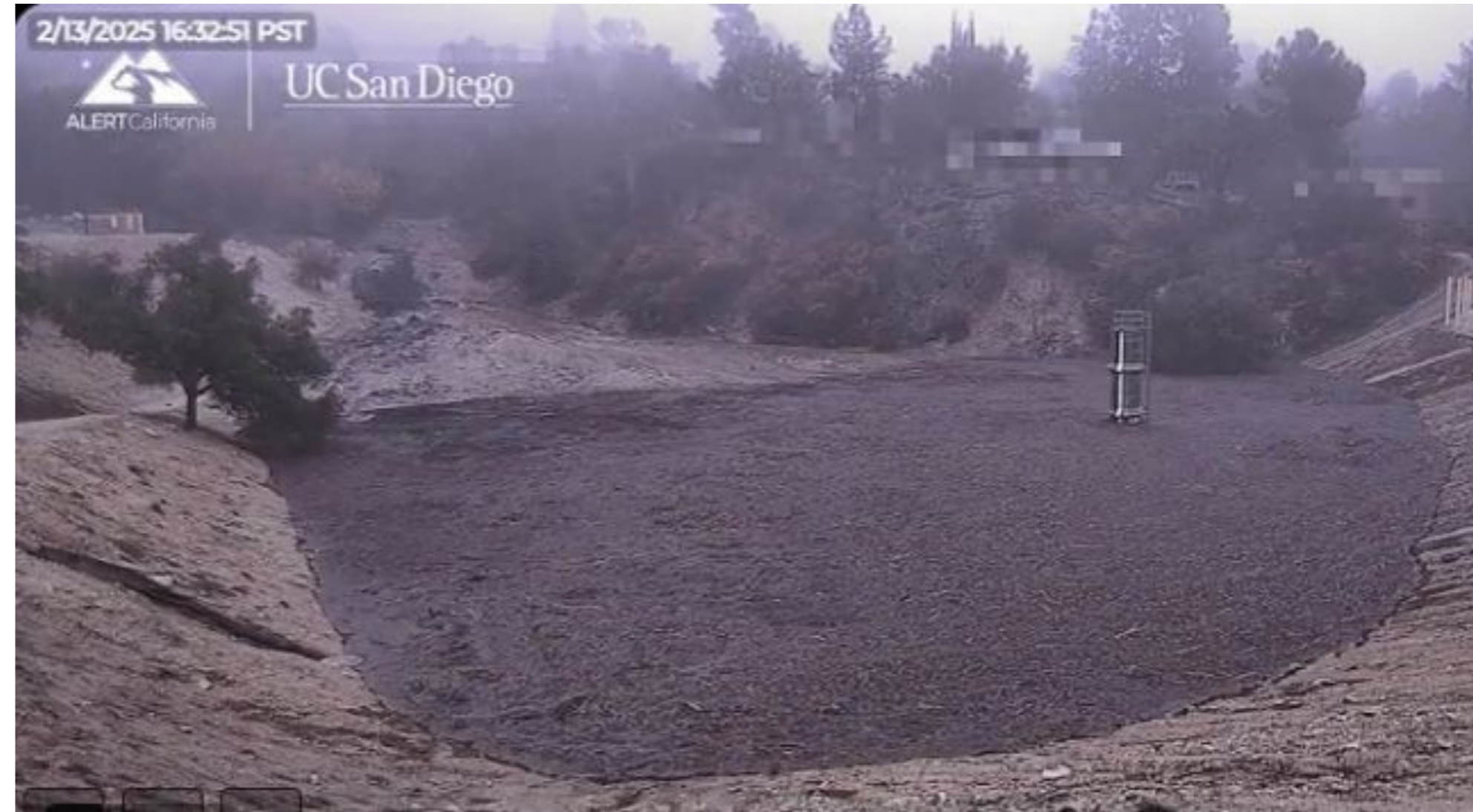
A debris basin in Bailey Canyon captures a significant amount of material which flowed from the Eaton Fire burn car
