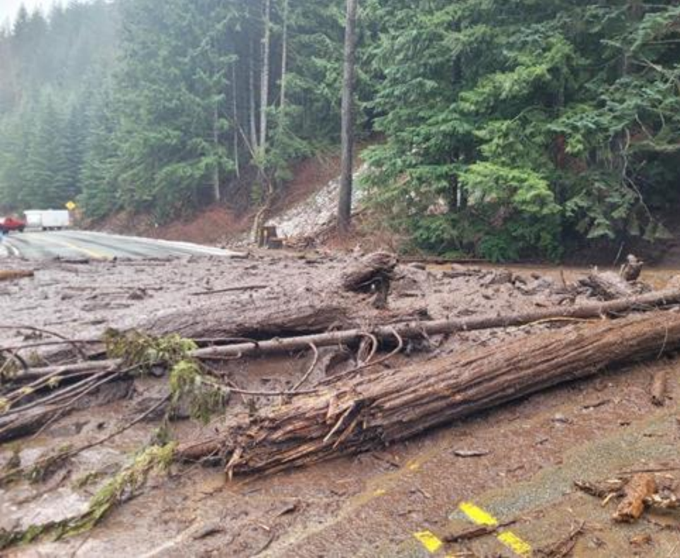
Landslide Across US 2 Near Stevens Pass, WA
