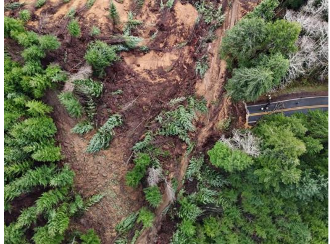
Landslide Across OR 229 North of Siletz, OR
